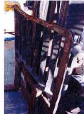
x Unacceptable damage to load guard
